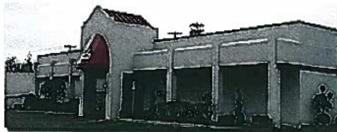
Buffalo Rheumatology received assistance to move from its Orchard Park location (top) to Sheridan Drive in Amherst (bottom), the former site of Fanny's Restaurant
