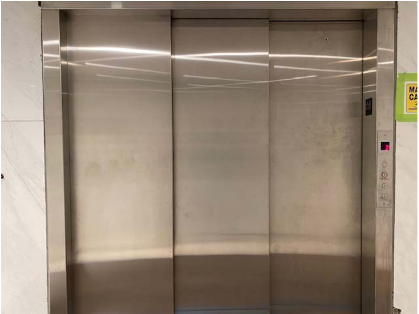
Our completely new high tech automatic freight elevator.
