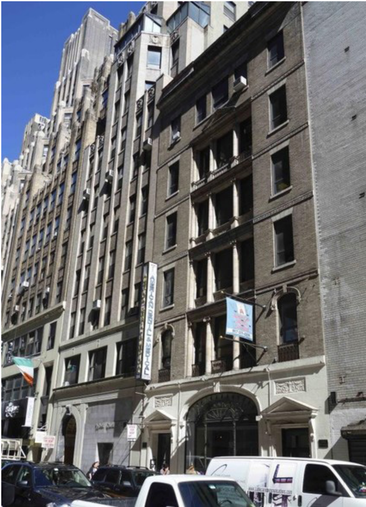
Farimont Building J.M. Heatherton, 1923 239-241 West 30th Street
