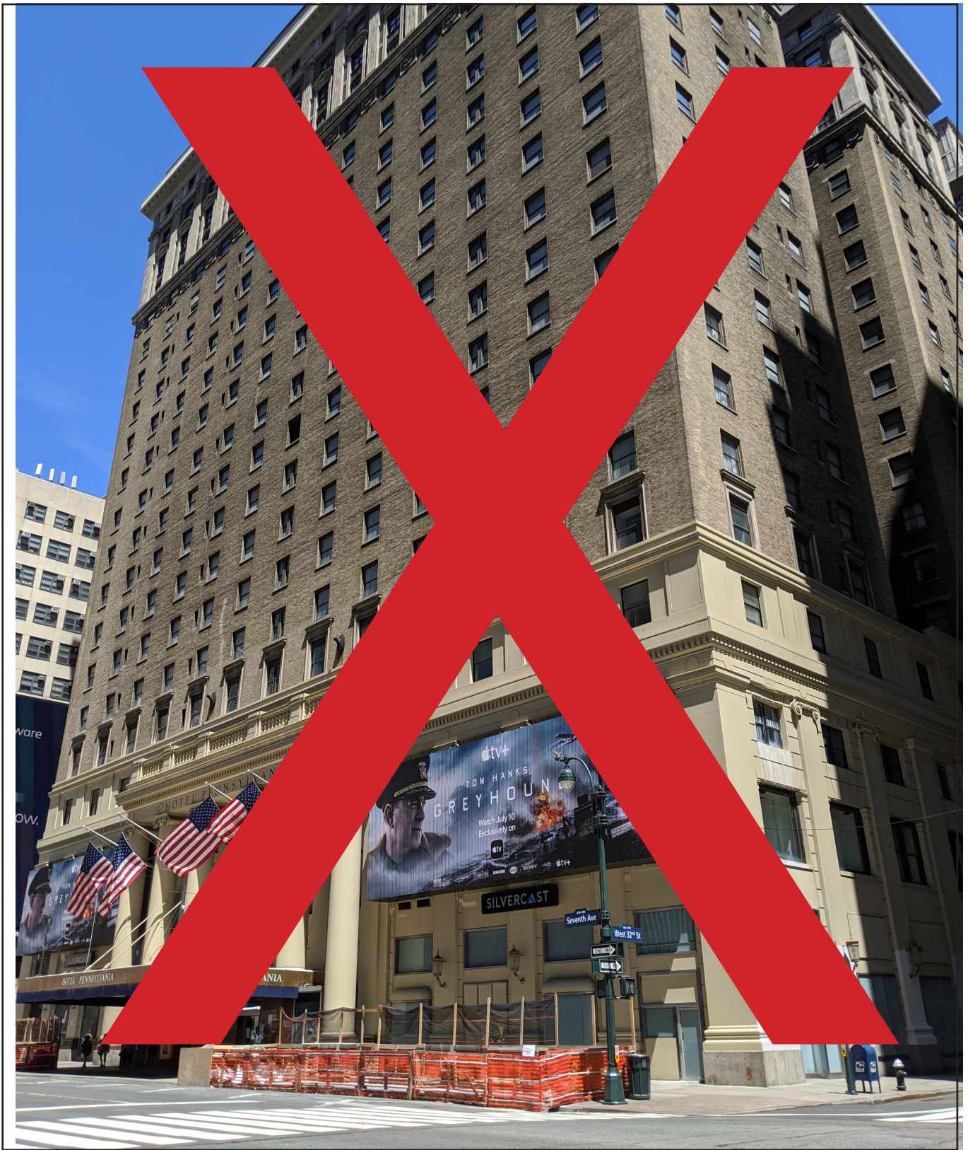
Hotel Pennsylvania Already being demolished McKim, Mead & White, 1919 401 7th Avenue
