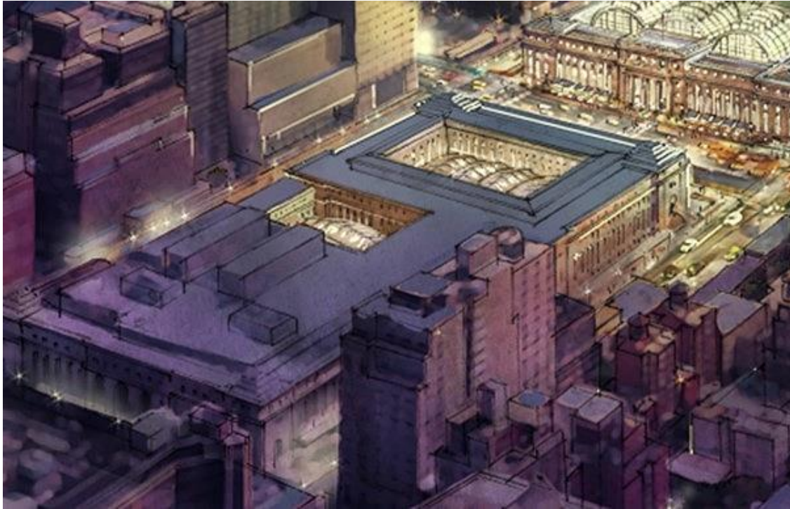
Moynihan Train Hall - Michael Evans Moynihan Station Project Lead - Rendering by Jeff Stikeman
