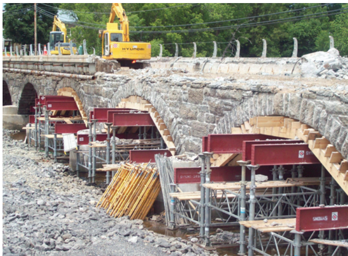
Bridge repair in Madrid NY. Photo courtesy of NYSDOT
