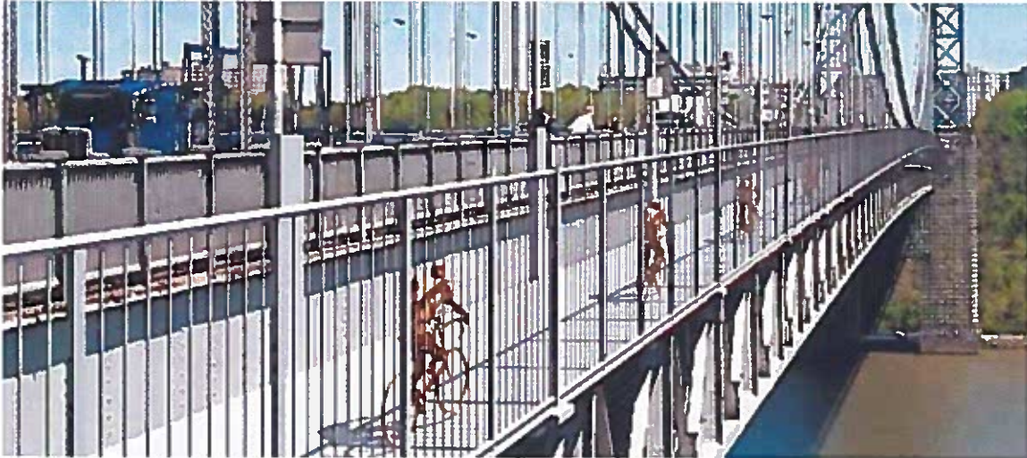
Complete George: (2) 10' paths for cyclists plus (2) 7' paths for peds-runners. 9' high anti-suicide barrier. Rendering Joseph Lertola.
